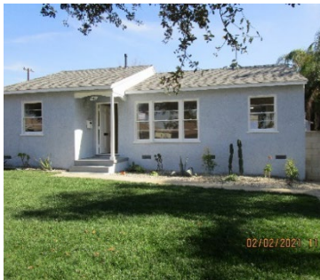
Code enforcement efforts leading to housing repairs.
