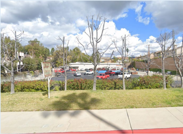
Site 17: Fire Sprinkler Shop
