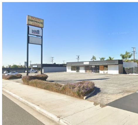
Site #14 at 2271 W. Whittier Boulevard
