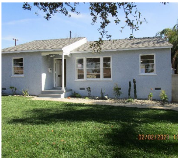
Code enforcement efforts leading to housing repairs.
